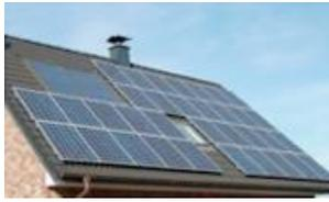
Solar photovoltaic (PV) systems convert daylight into electrical energy using a thin layer of semiconducting material, usually silicon. The potential electrical energy from a single PV cell is low, so cells are joined together to create a panel (or module). Panels are then joined together to create an array.
