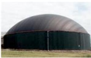
Anaerobic digestion (AD) is the process where plant and animal material is converted into useful products by micro-organisms in the absence of air. AD can accept waste from our homes, supermarkets, industry and farms, meaning less waste goes to landfill. The material is put inside sealed tanks and naturally occurring micro-organisms digest it, releasing methane that can be used to produce useful energy.
