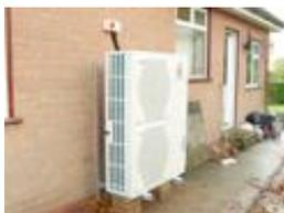
Air source heat pumps work in a similar way to ground source models but exploit the low level heat in the air rather than the ground.
